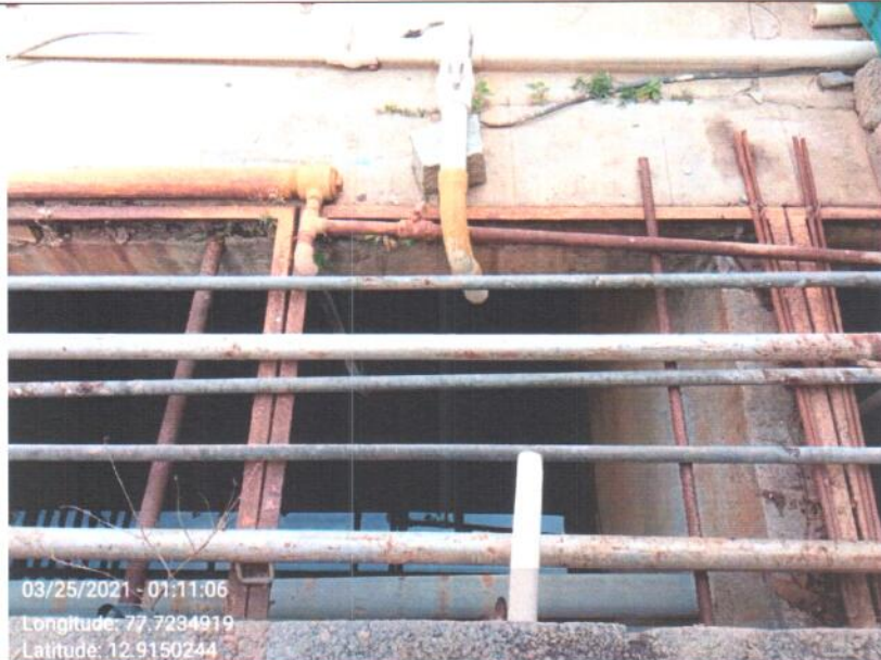
3rd tank after 1st time cleaning water come here for settling small particles
